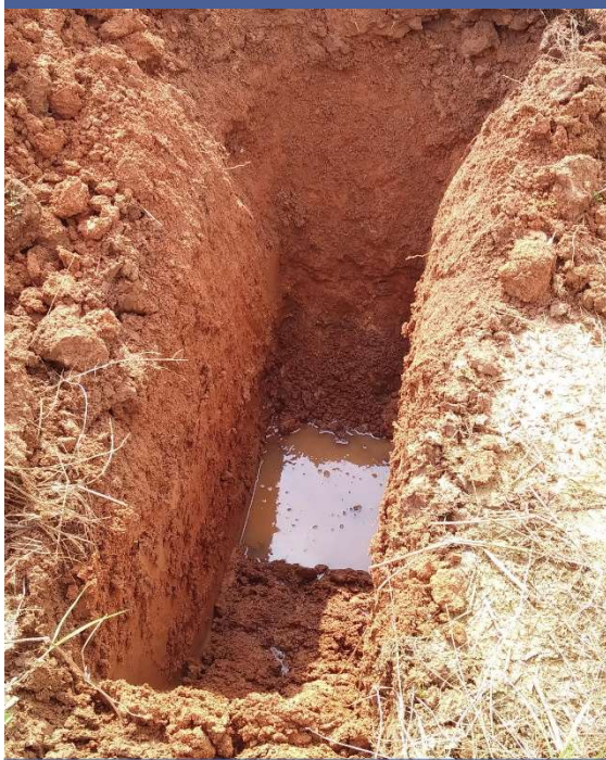
Trial pit showing the clay and shallow water table
